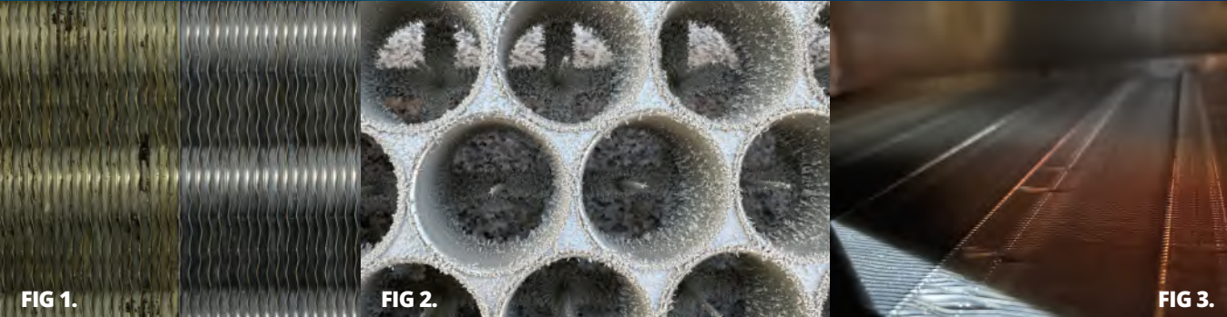
↑ FIG 1: The presence of biofilms on the cooling coils of commercial air conditioning (AC) units [FIG 1] can significantly reduce the heat transfer efficiency of the coils and may lead to the aerosolization of microbes into occupied spaces of a building.
